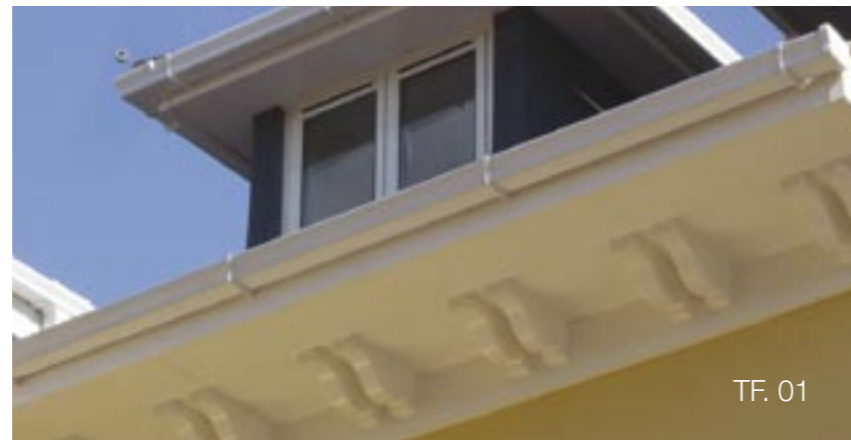
Typical Dentil Installation
